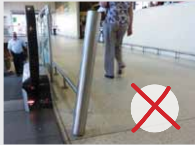
Traditional metal bollards do not absorb the impact.
