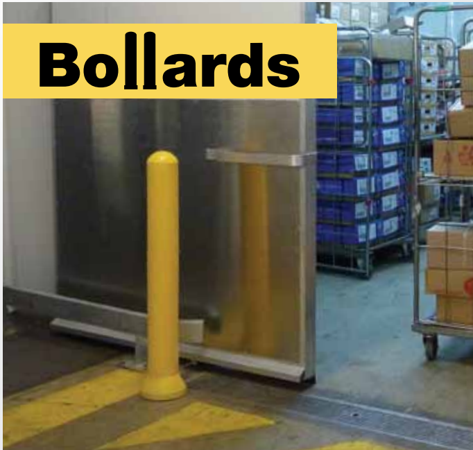
Traditional metal bollards do not absorb the impact.
